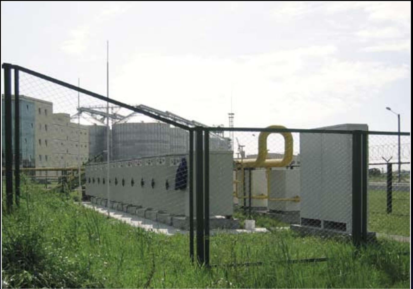
Example of installation of vaporizer cabinet units
